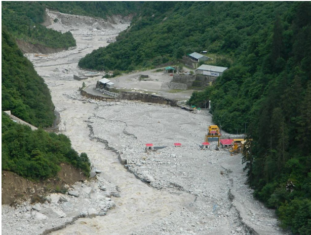
Vishnuprayag dam filled with boulders, the river bypassed the dam (Photo: Matu Jansanngathan)
